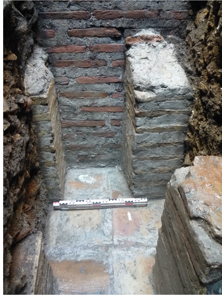
Suppl. Fig. 3. Detail of the hypocaust pilae against the north wall of room II, looking north. (B. Shkodra-Rrugia.)
