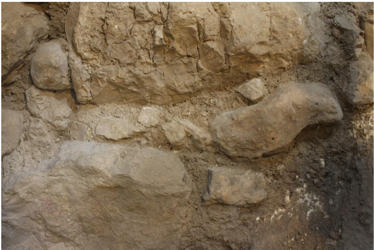
Figure S18. Area U: The “mud mortar” between the stones of wall, prior to sampling.
