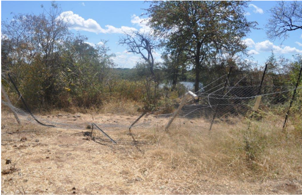
PLATE S2 A fence damaged by elephants in the A1 corridor through the Kasane community in Chobe District, north-eastern Botswana (Fig. 1). The fence was blocking the elephants from using the corridor and accessing the Chobe River.
