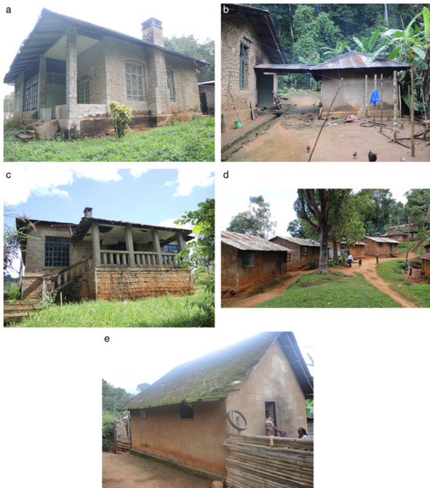
FIGURE 12A–E: Types of Amani housing stock: a German-built senior staff (forester’s) house, ca 1904; b Servants’ quarter and kitchen, attached to senior staff house, probably 1930s; c Senior staff bungalow, middle ridge, probably 1930s; d Junior staff housing, staff settlement, probably 1940s; e Junior staff housing, Market Street, probably 1950s.
