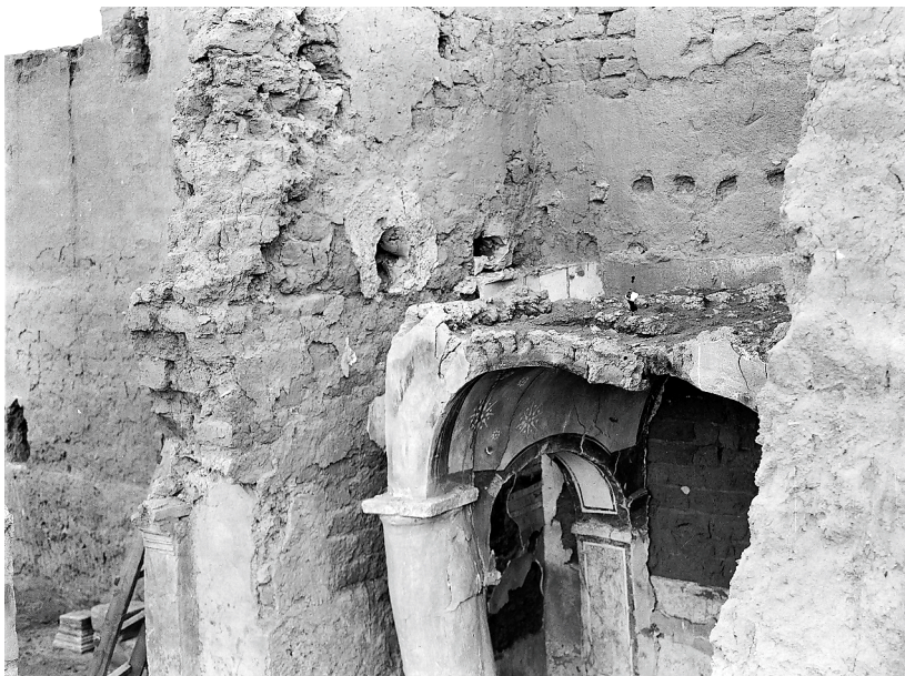
Suppl. Fig. 1. Photograph of the south end of the canopy of font in Room 6, showing joists of later ceiling. (Dura-Europos Collection, YUAG, neg. Dura-I682b-01, courtesy YUAG.)
