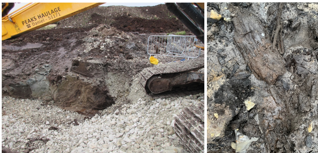
Figure S1. Left: Excavation of deposit, right: large wood fragments excavated
